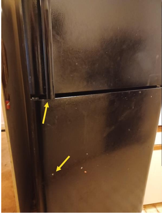
Refrigerator door handle broken off. Arrows show where mounting holes are located.
